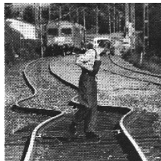
(Left: Buckling due to glaze icing; Right: Buckling of rails)
